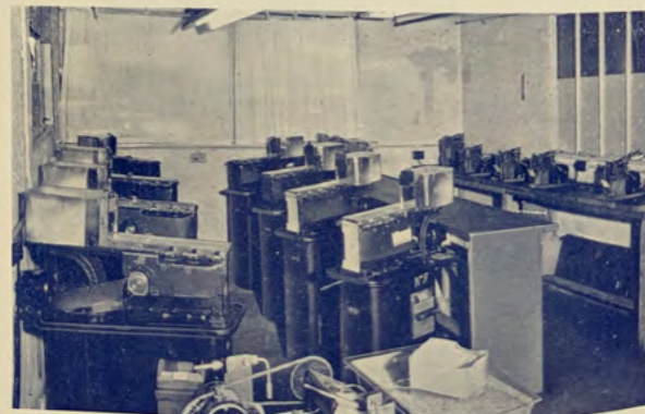
Fig. 5. Works-designed apparatus is employed for the grinding of balls automatically. machines in the foreground for the larger sizes, those in the background being for sizes of 1 mm. and under. The machines gauge to a tolerance of 0.00002 in.
